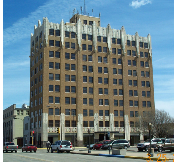
United Life Building, 119 W. Iron Avenue
