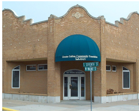
Awning accentuates the main entrance to a building.
