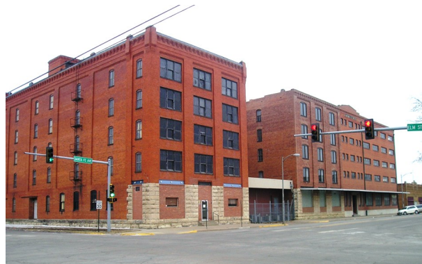
248-254 N. Santa Fe Avenue, H.D. Lee Complex
