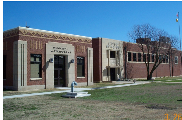
City Water Treatment Plant, 401 S. 5th Street
